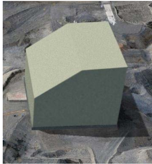
Figure F.3-6. Interim Safe Storage Enclosure
